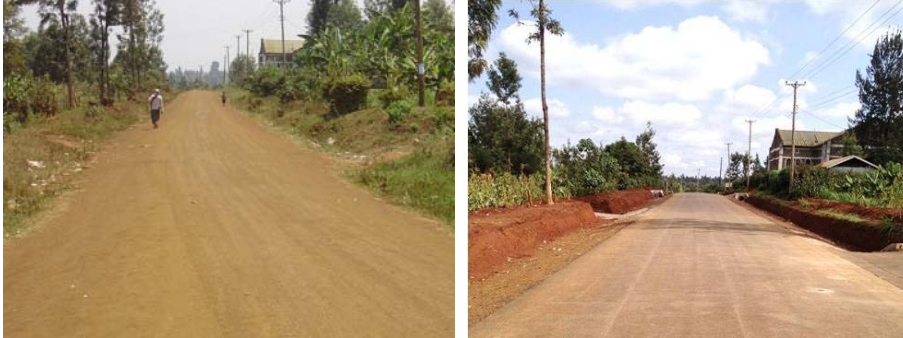
Figure 3: Example of widening from 4.5 m to 6.0 m
