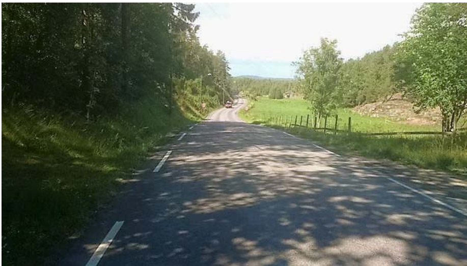
Figure 1: Low volume rural road in Norway, 5.50 m wide with AADT 2000
