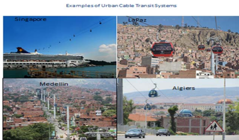
Fig.2. Typical ropeway installations
