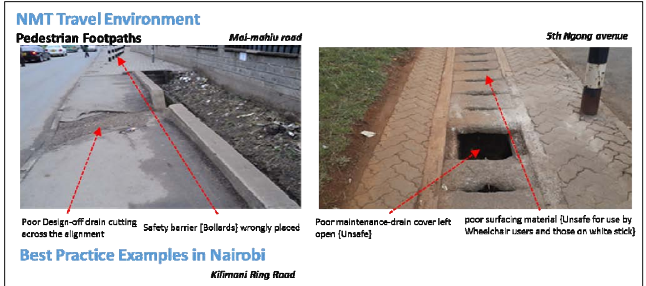
Figure 3-1: Picture of a poorly designed and maintained sections of a footpath in Nairobi city
