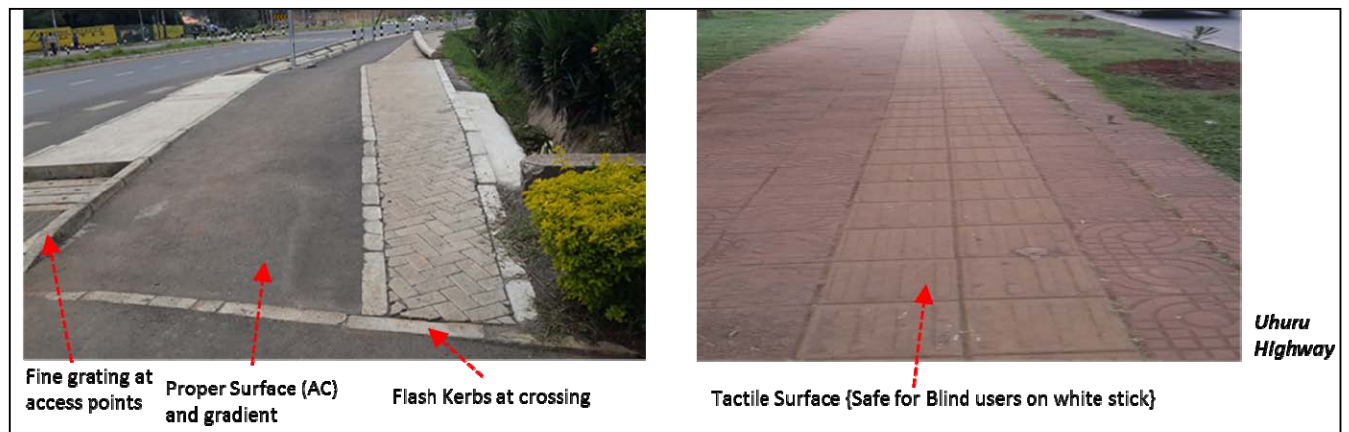
Figure 3-2: Picture of a well-designed section of a footpath in Nairobi City
